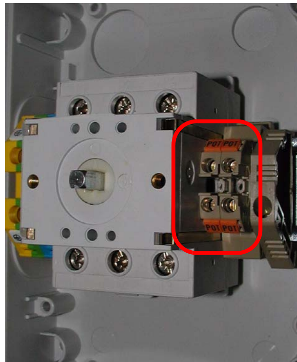
Fig. 5-2: Main switch, POT-kontakt
